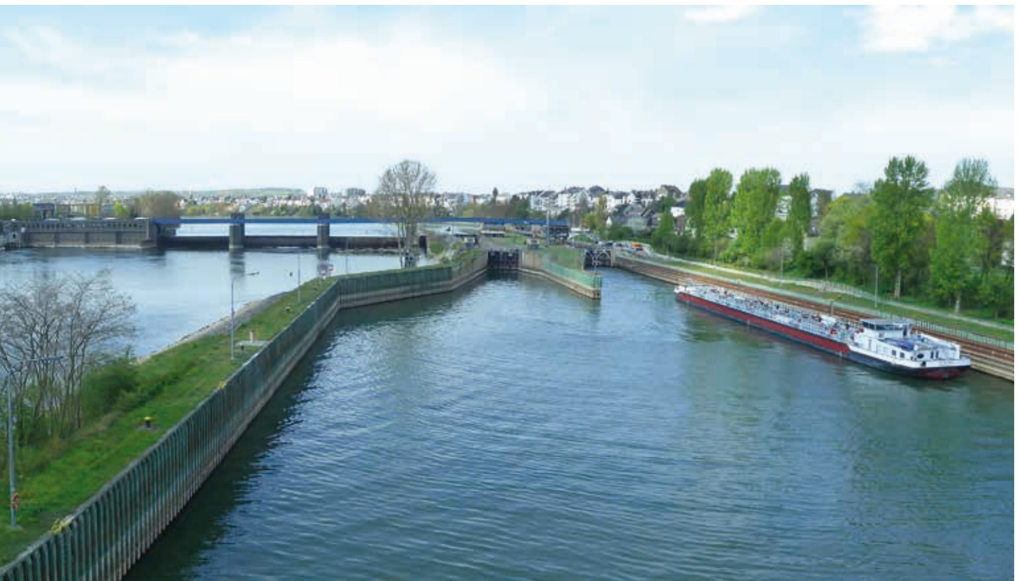
Koblenz barrage weir in the Moselle; urban development, transport infrastructure, hydropower use and navigation determine river engineering measures Source: Stephan Naumann
