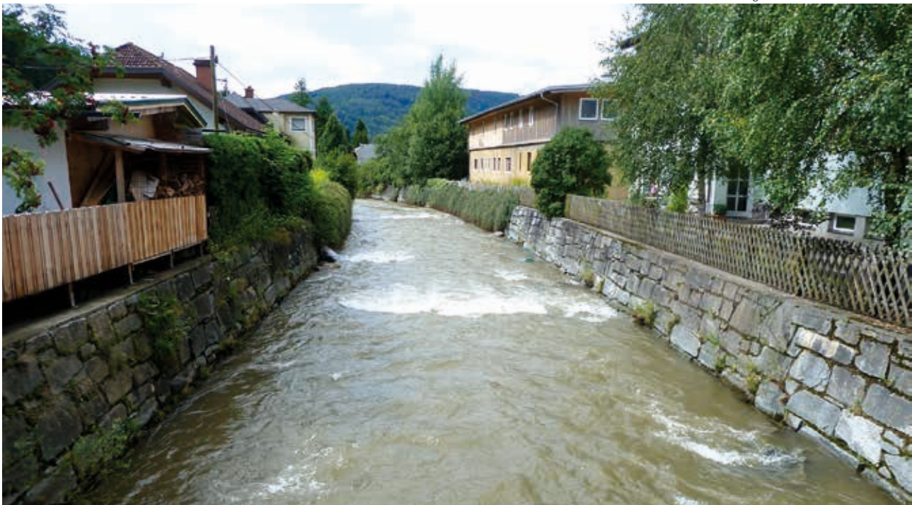
River in the Central German Highlands developed for flood protection Source: Stephan Naumann
